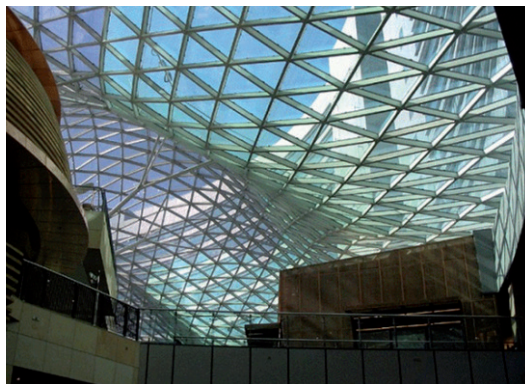
Roof of Zlote Tarasy atrium (Golden Terraces) in Poland. Waagner-Biro GmbH, Austria, winner of the European Award for steel construction 2007
