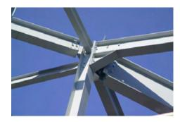
Steel connections detailing software as well as the standards worldwide, are dealing only with typified connections. In real life this is not a certainty. There are many times when the engineer must evaluate the strength of complicated connections by dividing them in smaller components - well described in the standards – and examining each one of them.
